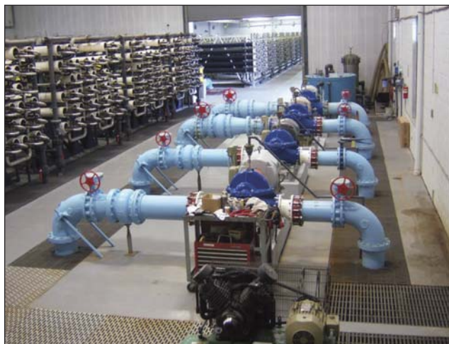
Figure 5. View of membranes in use at the reverse osmosis plant in Cape Coral. (photo: Hubert Stroud)
