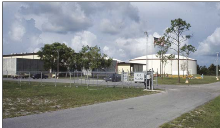
Figure 4. Ground view of reverse osmosis plant at Cape Coral. (photo: Hubert Stroud)
